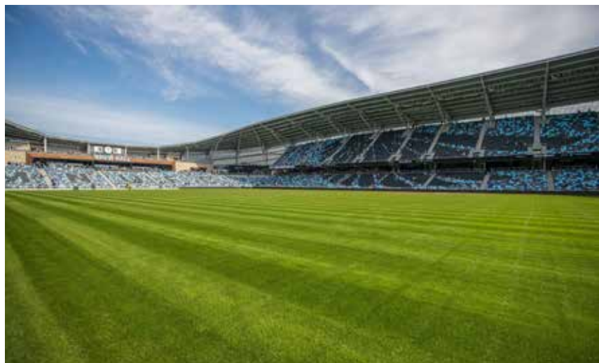
A hydronic field heating system and high capacity drainage system keep the pitch match ready.
