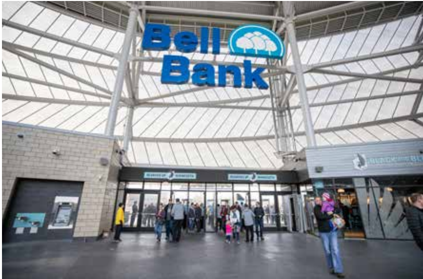
The Bell Bank gate, on the southwest side of the stadium, is highly visible from the highway.
